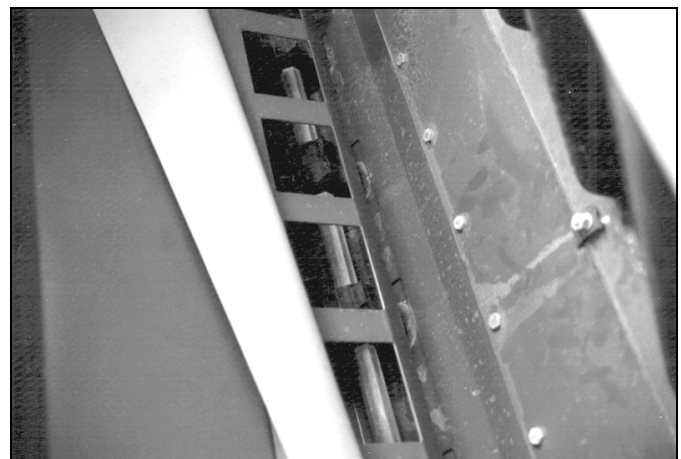
Figure 96 Dew Shield at Openings
