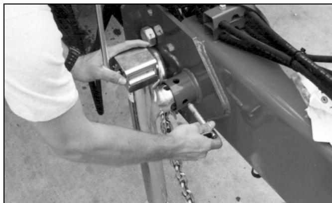
Figure 4 Jack in Lifting Location
